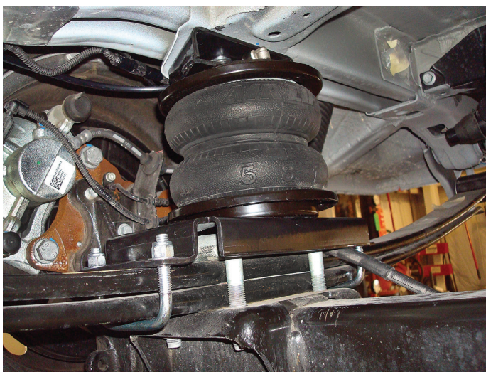
Front view of the passenger's (right) side installation.
