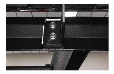
**Step 7:** After finial adjustment, tighten all hardware starting with the three lower bolts and then finish with the upper bolts.
